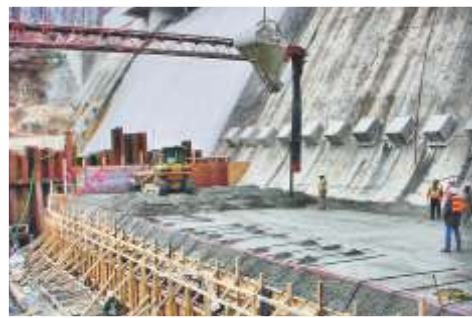
DAM REINFORCEMENT 50,000 CY OF ROLLER COMPACTED CONCRETE
