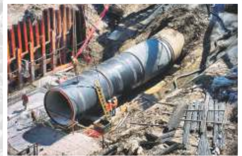
120" DIAMETER PRE-STRESSED CONCRETE CYLINDER PIPE REPLACEMENT
