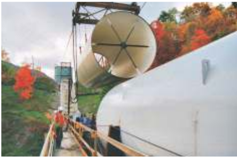
WATER CONVEYANCE PENSTOCK HIGH LINE INSTALLATION
