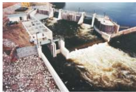
CONCRETE FISH PASSAGE CONSTRUCTION
