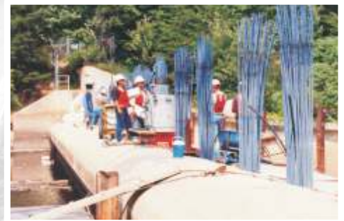
ROCK ANCHORING OF DAM
