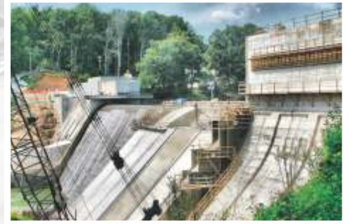
125 FT HIGH GRAVITY DAM REHABILITATION
