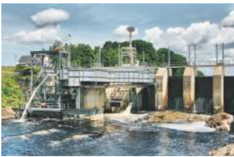
FISH LIFT SYSTEM STEEL FABRICATION INSTALLATION
