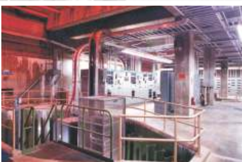
NEW CONTROL ROOM CONSTRUCTION
