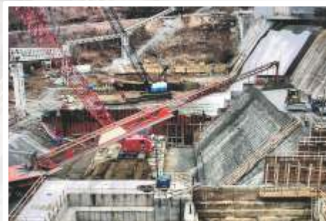
DAM STRENGTHENING & REFACING
