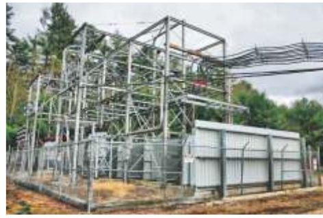
SUBSTATION CONSTRUCTION / UPGRADES
