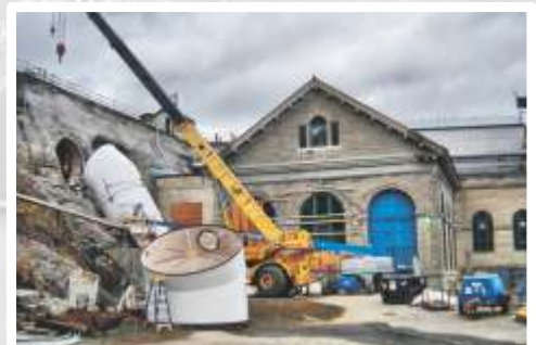
STEEL PENSTOCK REPLACEMENT
