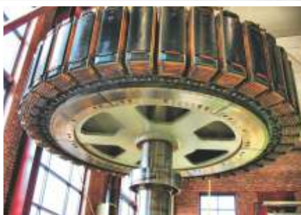
TURBINE ROTOR INSTALLATION
