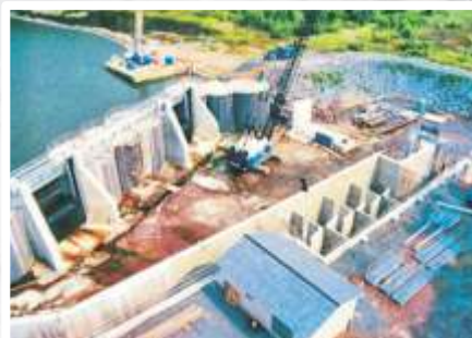
DAM / GATES / FISH PASSAGE INSTALLATION
