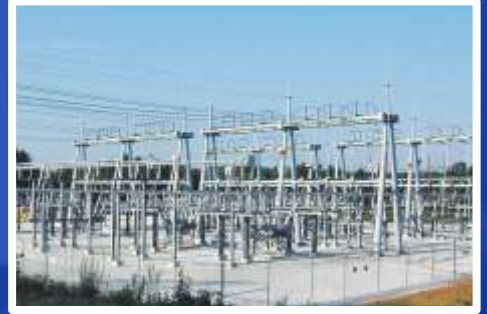
345 / 115 kV SUBSTATION
