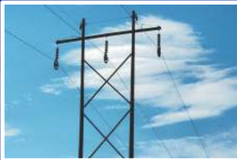
115 kV SECTION REBUILD
