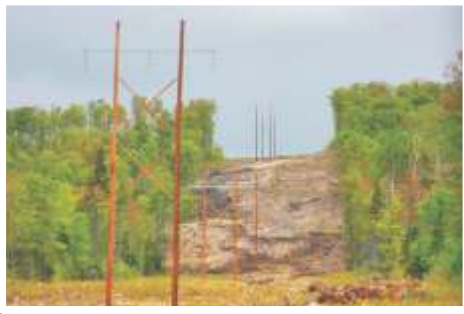
27.2 MILES - 115 kV TRANSMISSION LINE
